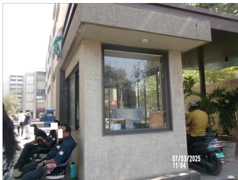
Security room - Main building
