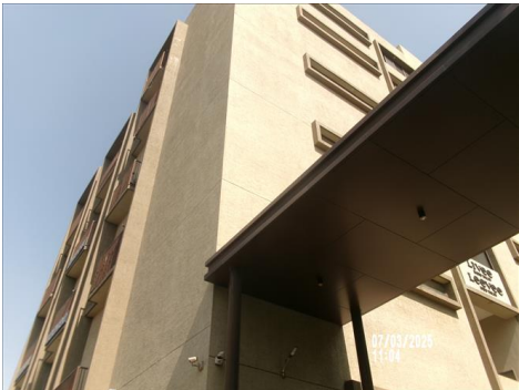
Overview of facility
