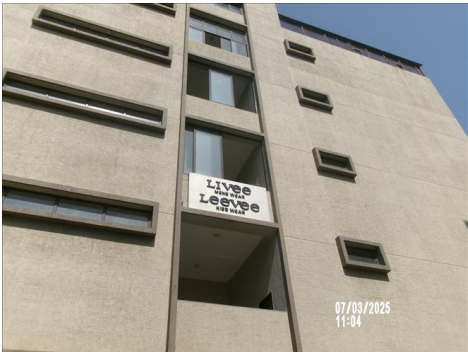
Overview of facility
