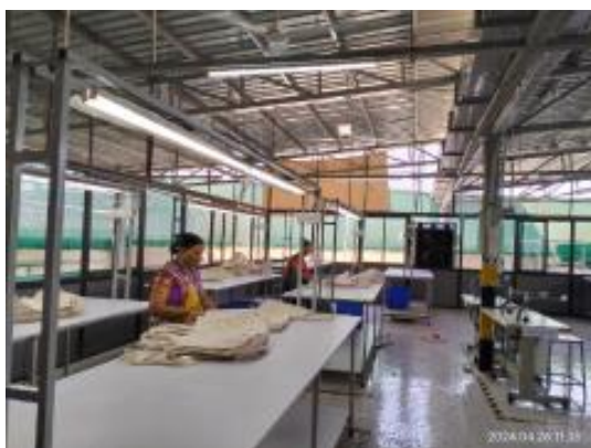
Air Cooler provided in first floor.jpg
